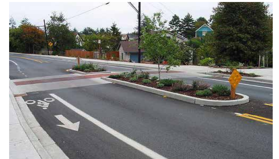
Reflectors and slightly raised crosswalk
