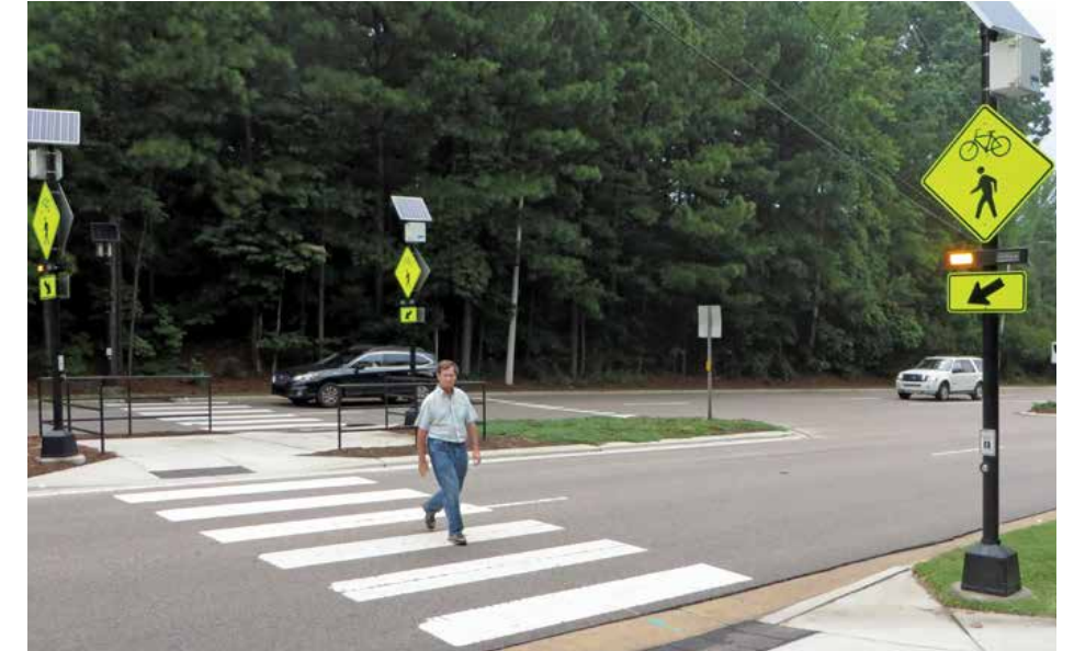
Flashing beacons and medians can help improve pedestrian safety
