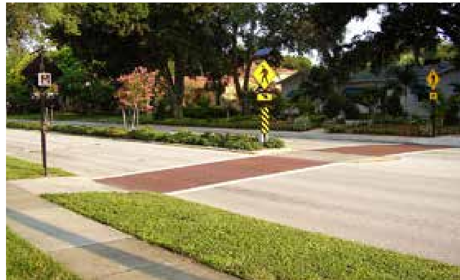
Brick pavers and flashing signage clearly alerts oncoming traffic
