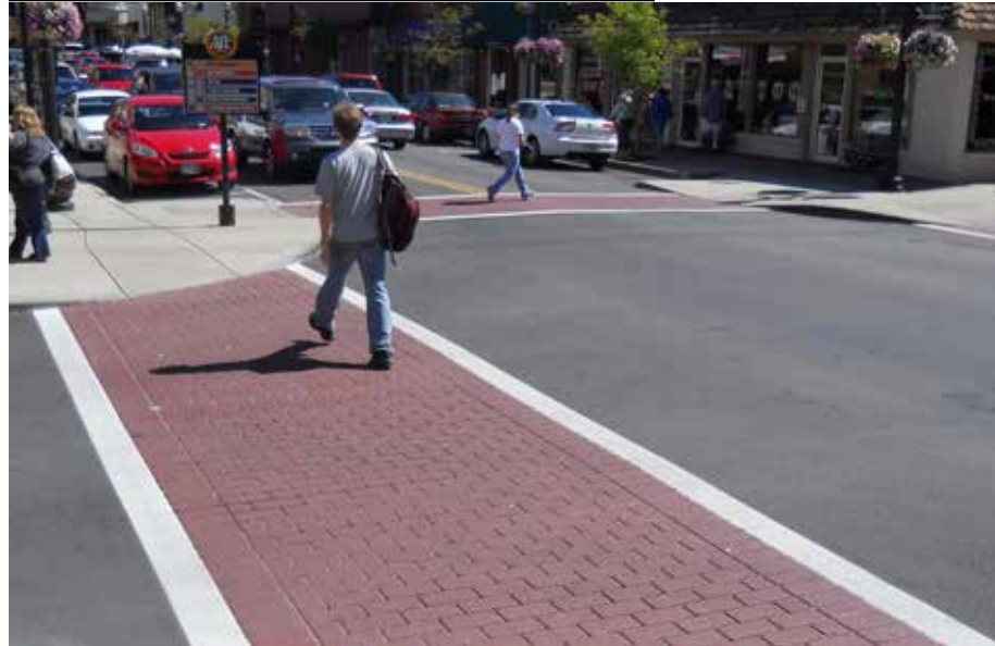
Brick pavers can be used to clearly delineate the crosswalk.
